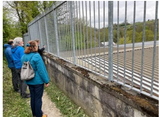
Figure 4 - Twigg Stores roof from the footpath
